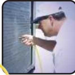
Blow off coils with Blowgun
