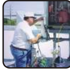
Purge and pressure test an A/C&R system
