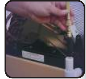
Clean out condensate drain lines with Sludge Blaster®
