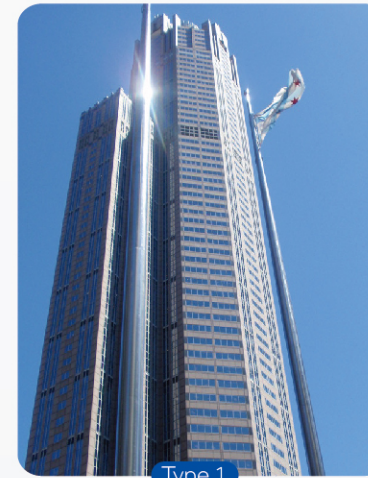
High rise building without podium
