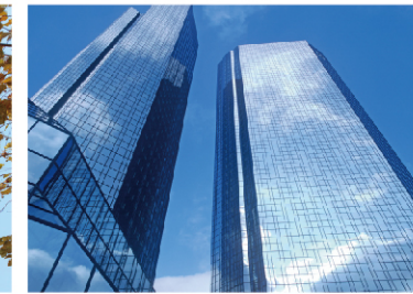
High rise building with podium
