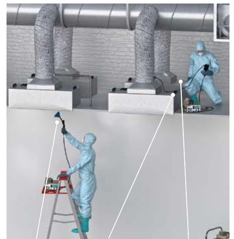
Leak testing with a photometer or DPC
